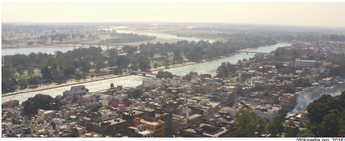
Figures 1- 3: Haridwar demo site for bottom entry well
